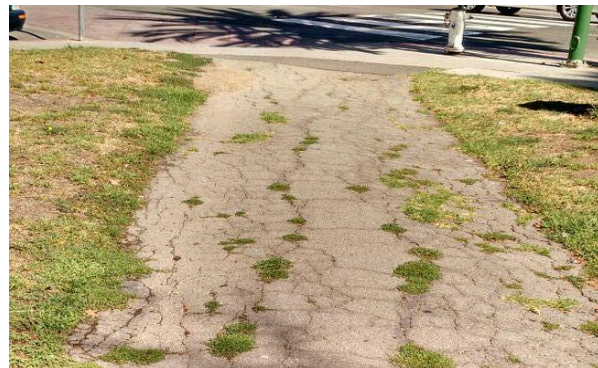
Clinton Square walkway
