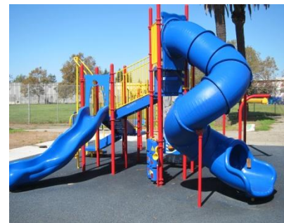
Wade Johnson-Resilient surface is in good condition.
