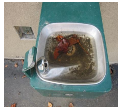
Poplar-leaves plugging drain.
