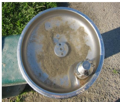
Verdese Carter—Sand plugging drain
